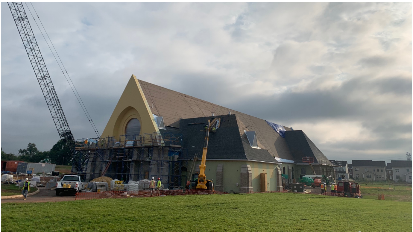
VIEW FROM SOUTH WEST CORNER
