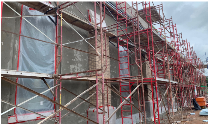
STUCCO AND GRANITE INSTALLATION AT NORTH ELEVATION
