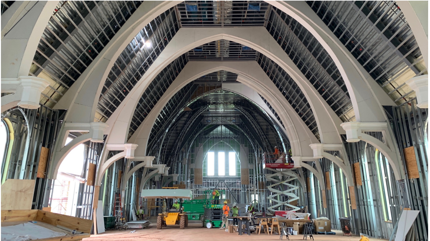
DRYWALL AND CANAMOULD AT NAVE ARCHES FACING EAST
